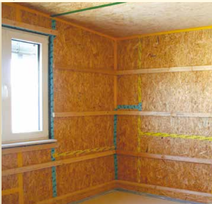
Airtight connections between wood composite boards
