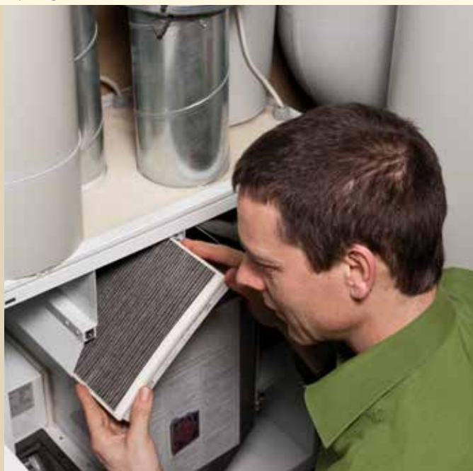
Replacing the filter of a ventilation unit.
