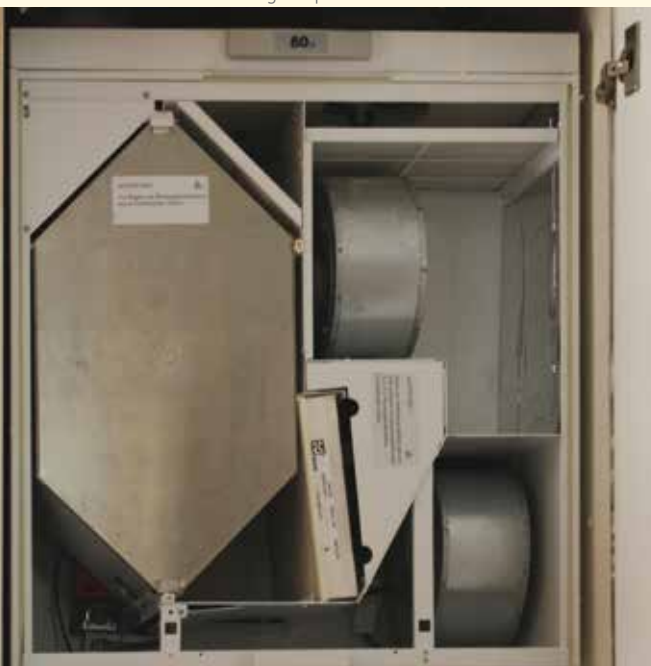
Ventilation unit with heat exchanger exposed
