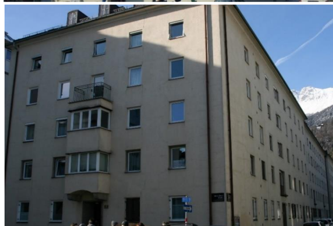
This apartment building in Innsbruck received not only good thermal insulation but also an extension as part of the SINFONIA refurbishment (view below before refurbishment). © Passive House Institute
