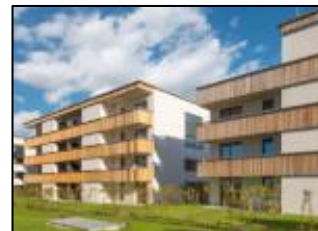
Socially compatible and highly energy efficient apartment blocks built to the Passive House standard. © Neue Heimat Tirol
