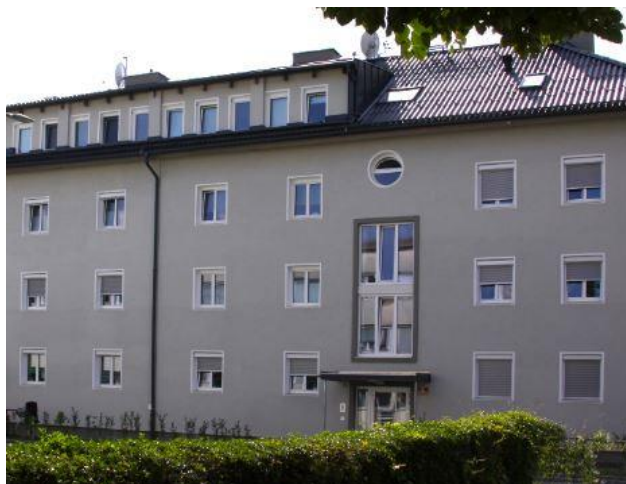
Innsbruck: Visitors can view this apartment block retrofitted by the housing association Neue Heimat Tirol to the EnerPHit standard. ID 5673 © PHI
