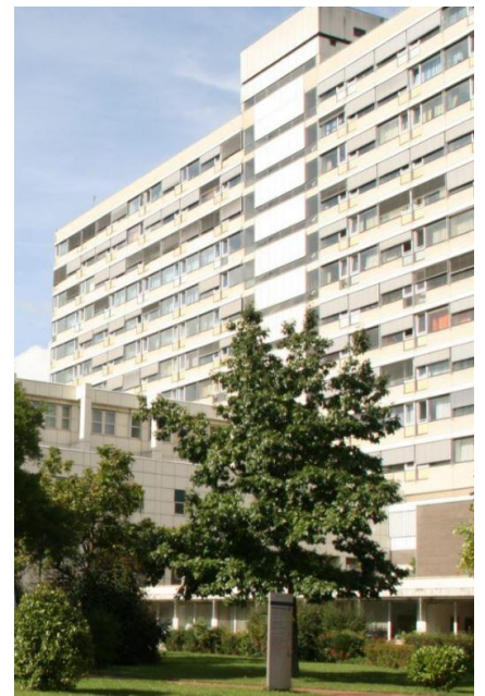
The existing hospital building in Frankfurt which was built in the 1960s. © Klinikum Frankfurt Höchst
