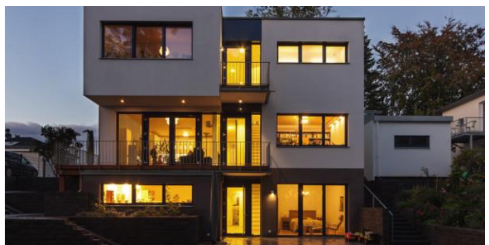
Passive House in Berlin with renewable energy and utilisation of rainwater. © Andrea Kroth
