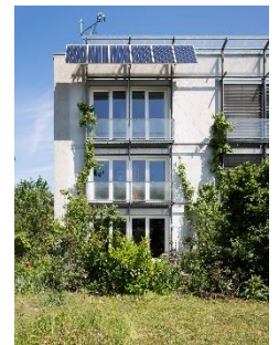
The world's first Passive House in Darmstadt-Kranichstein. © Peter Cook
