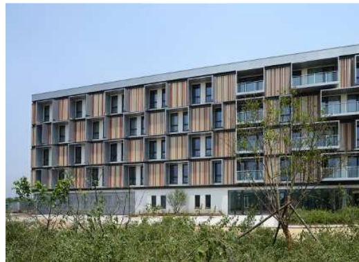
Fixed shading elements provide protection from too much sun. Photos: Peter Ruge Architekten / Jan Siefke
