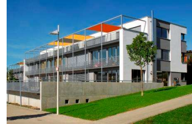
Row house with common underground garage in Ulm, Germany; © Casa Nova, Planungs- und Wohnungsgesellschaft
