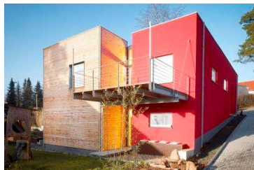
Single family house in Kaiserslautern, Germany; © Franz Josef Zimmermann, Planschmiede
