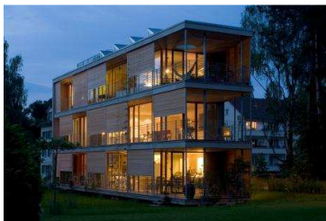
Multifamily building in Liebefeld, Switzerland (external view); © Peter Schürch, Halle 58 Architects, Bern
