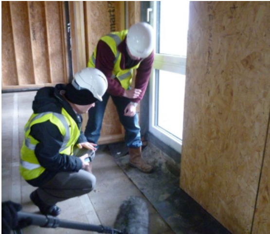
A visit to a Passive House construction site in the town of Fulmodeston in Eastern England.
