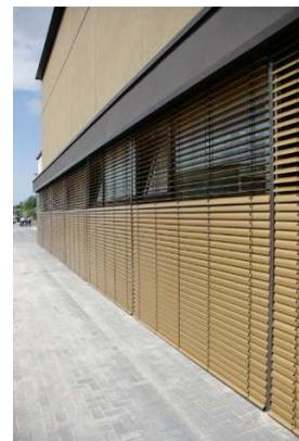
Detailed view showing shading elements.
